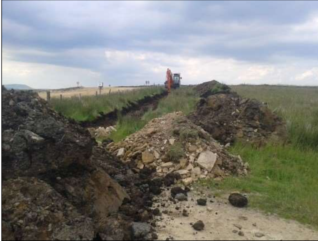
Figure 2 - Stockpile and drainage ditch (under construction)
