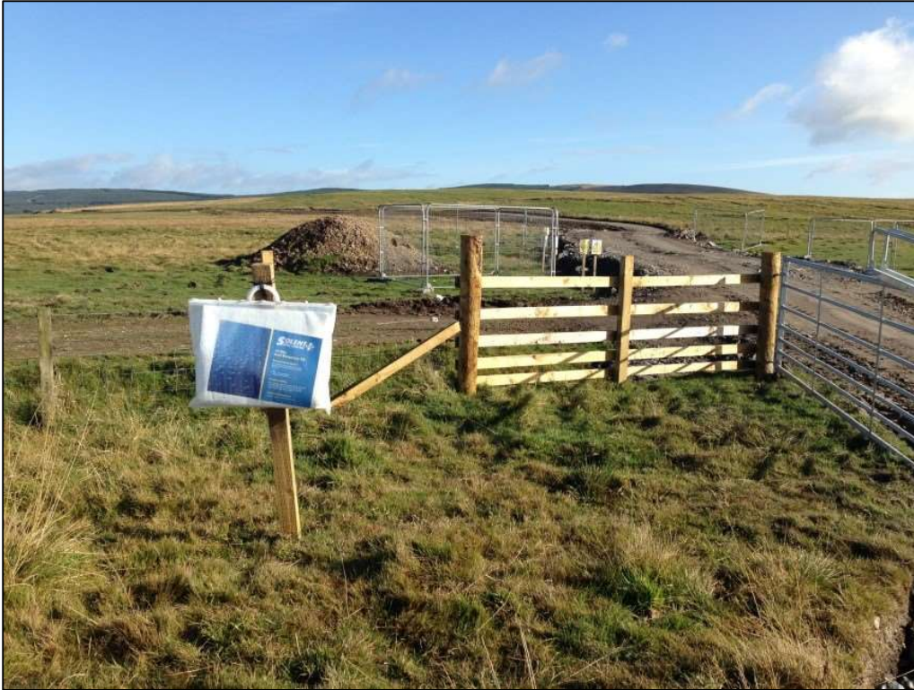
Figure 9 - Spill Kit Provision on Site
