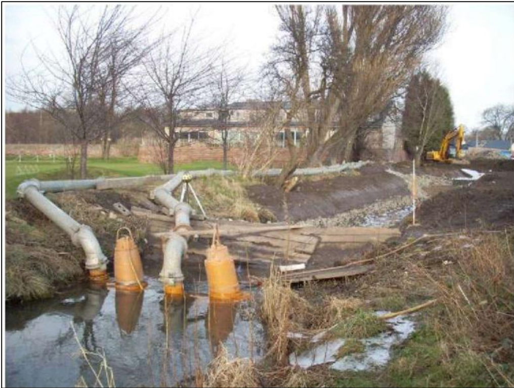
Figure 14 - Watercourse Diversion (Full Isolation - Over Pumping) 41
