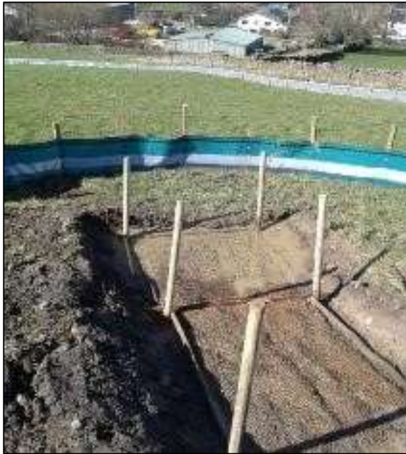
Figure 3 - Silt Matting (combined with silt fencing)
