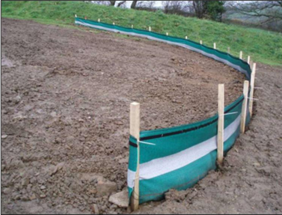
Figure 4 - Typical Silt Fencing
