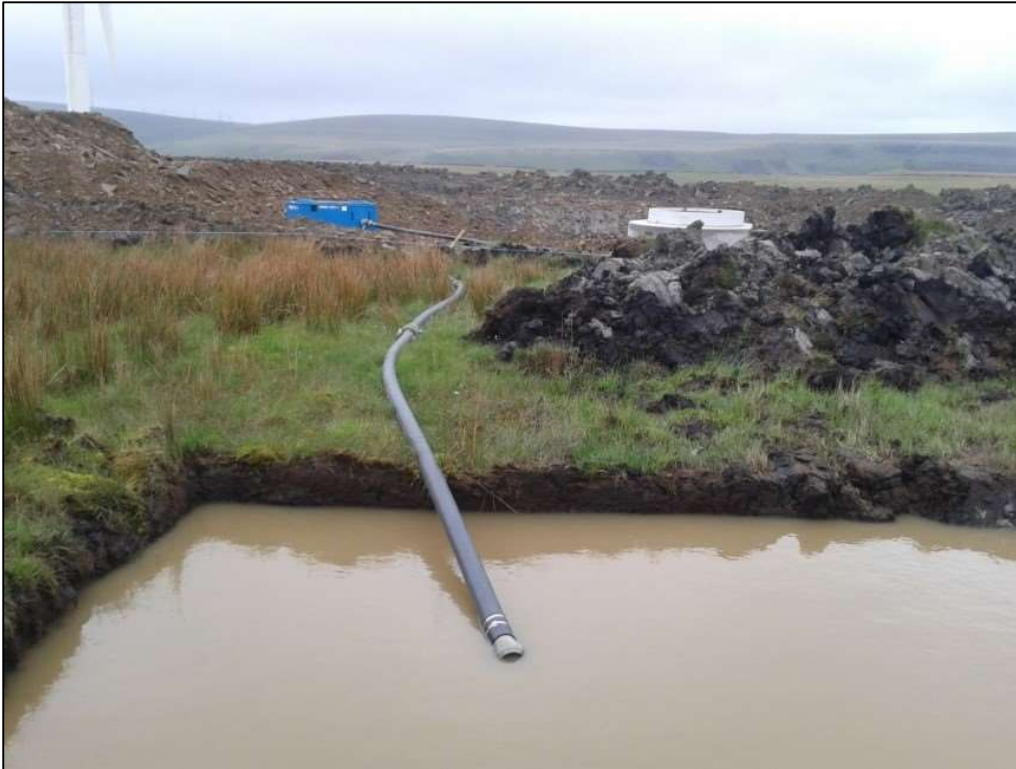
Figure 8 - Settlement Lagoon and Siltbuster Pumping Water for Treatment
