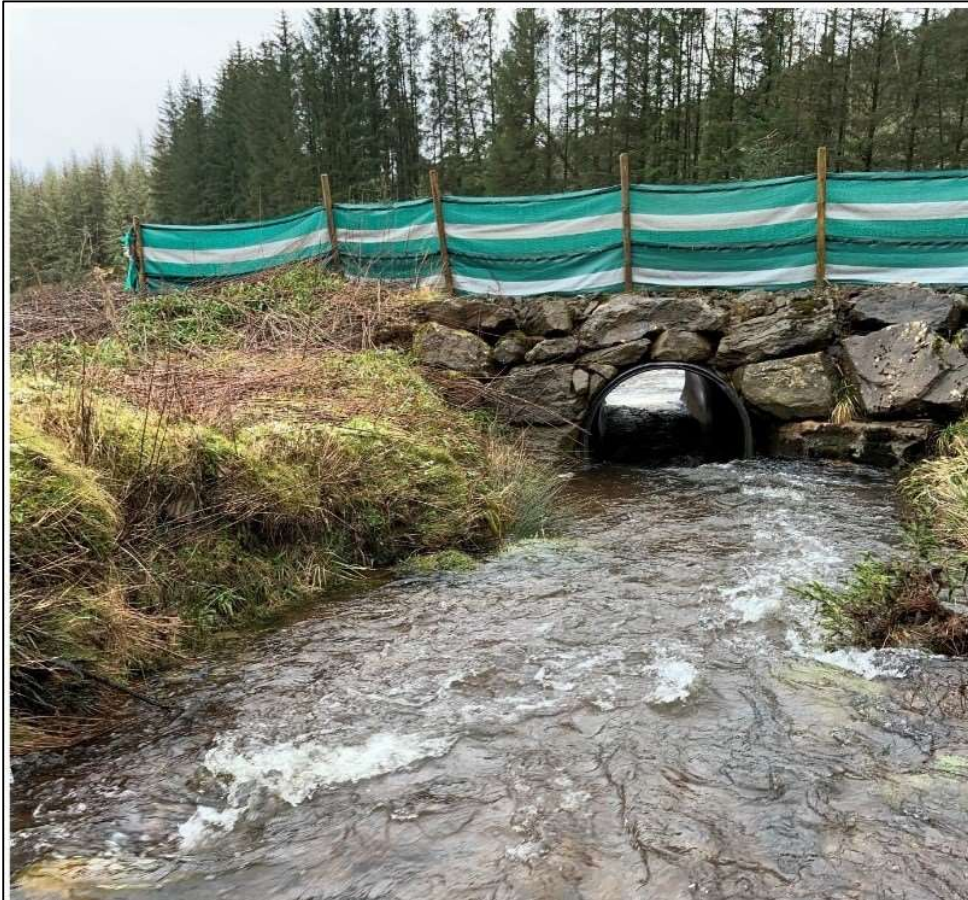
Figure 5 - Silt Fencing at Watercourse Crossing
